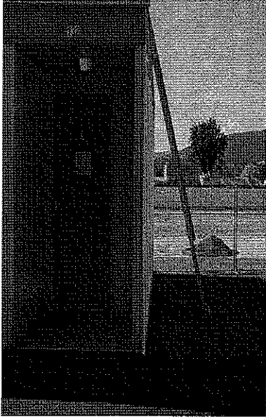
Proper 4 to 1 set-up outside a portable
