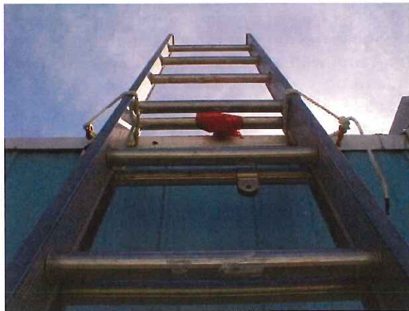
Best Practice Note: Tie-offs with separate nylon ropes to eyebolts left & right.
